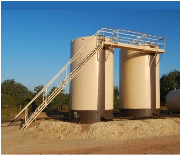
Twin 210 barrel oil tanks inside containment dike
